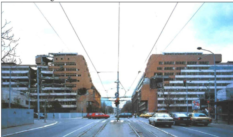
Fig. 4. The Army Headquarters after the 1999 bombardments and redefined recognisability. The Building A with significant damage and the Building B with slight damage and demolished entrance pavilion (on the far right)
